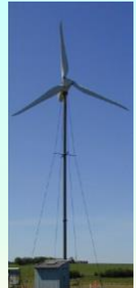
Guy-wired pole tower
