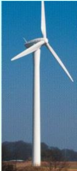
Tubular steel tower
