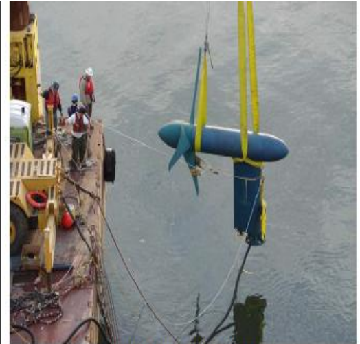
Figure 21: Free Flow Turbine Courtesy of Verdant Power
