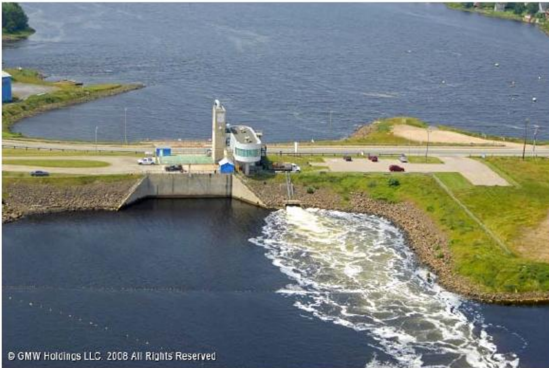
Figure 6.15: 20 MW tidal power plant at Annapolis Royal, Nova Scotia, Canada. TSU
