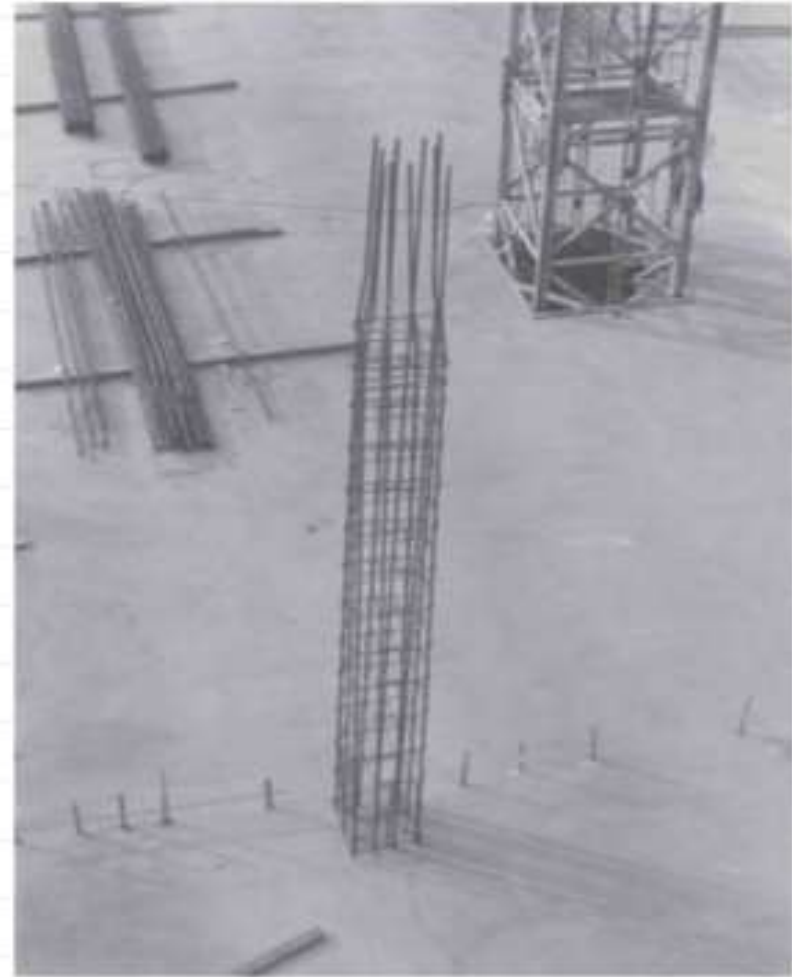
Reinforcement cage for a tied column
