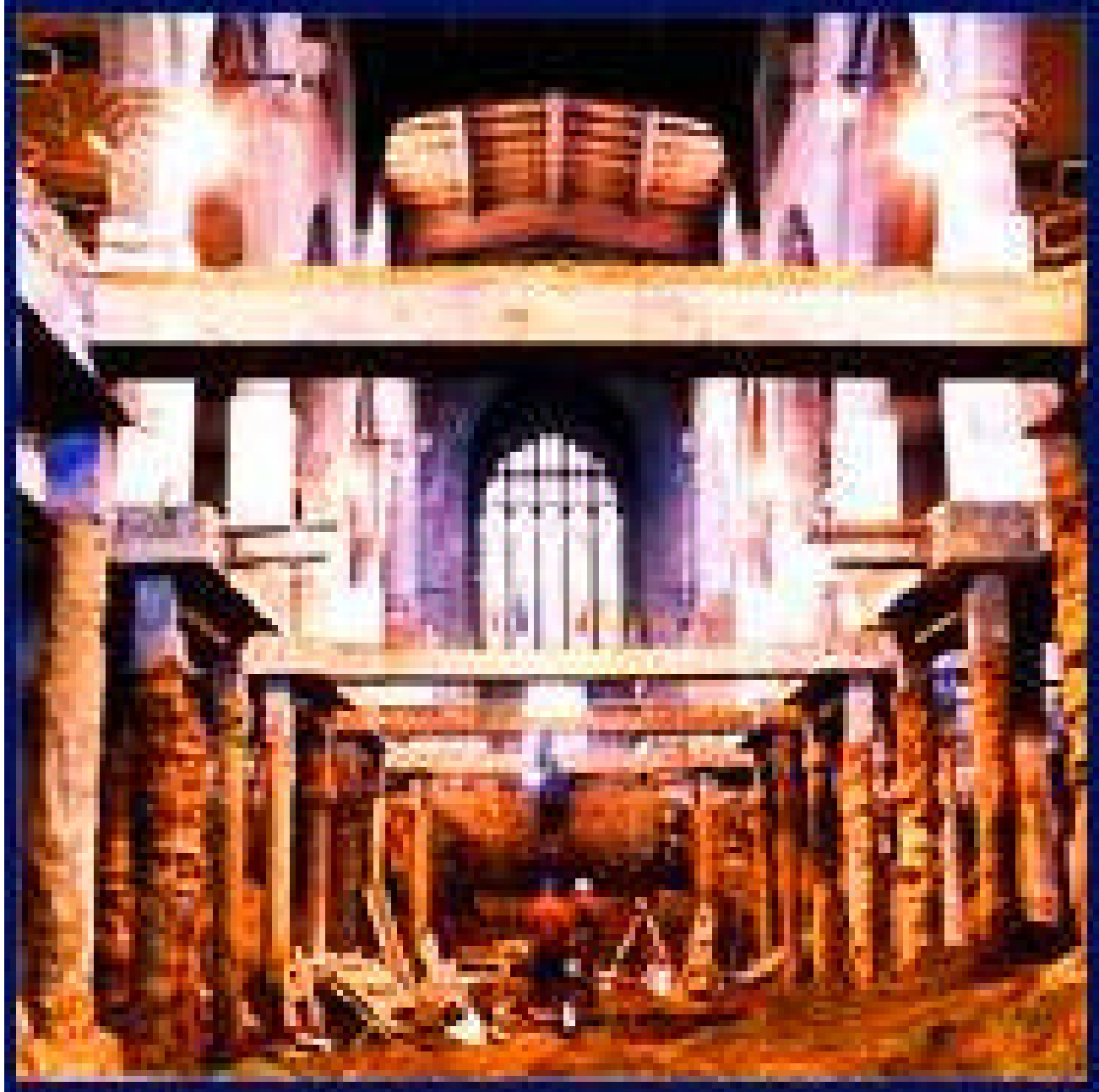
The ancient church of St. Nicholas, Sevenoaks, Kent, used mini piles to underpin the 800 year old church to support the building whilst providing a new undercroft.
