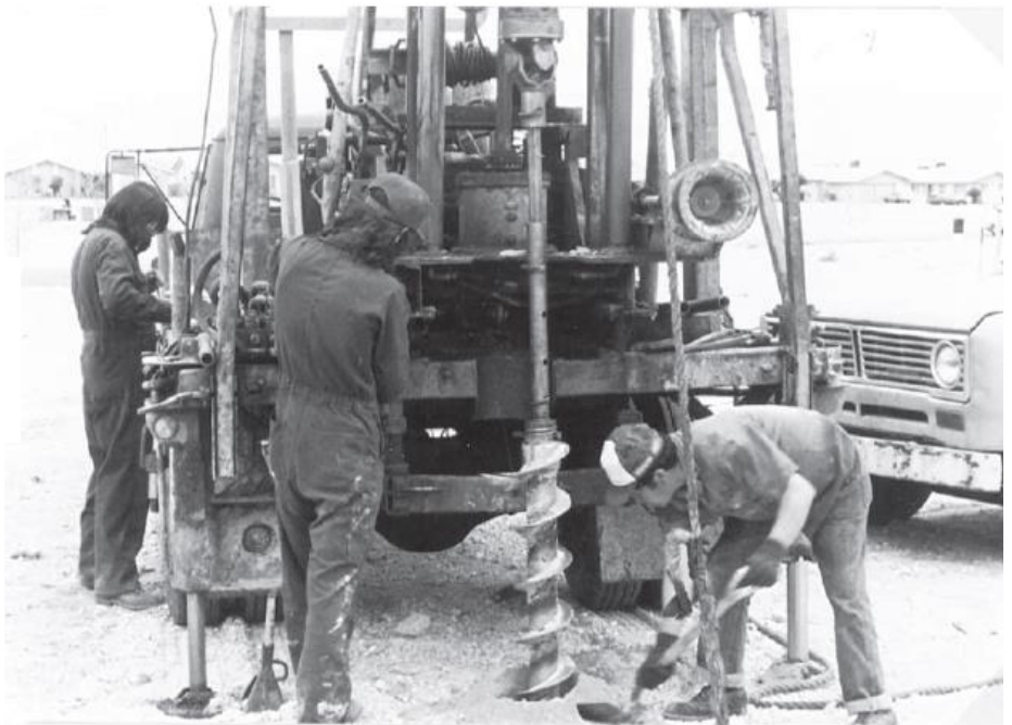
Figure 3-3 Soil drilling using a continuous-flight auger.
