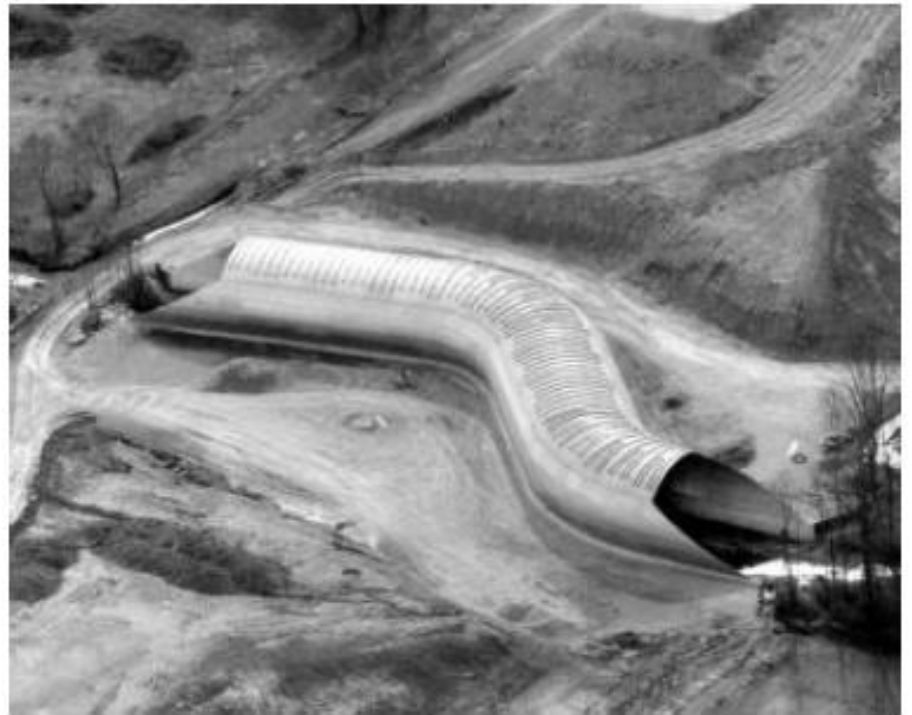
Figure VI-4--Culvert with a Horizontal Bend (Contech)
