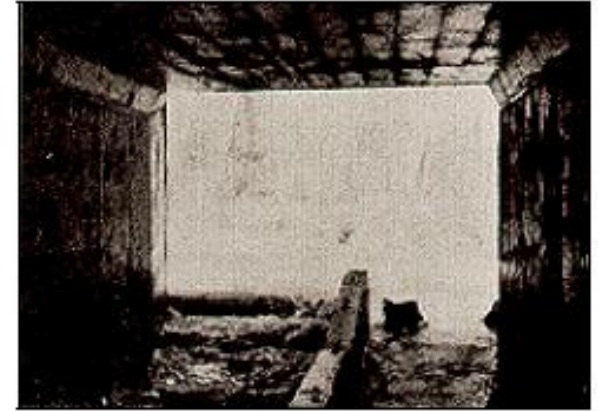
Figure VI-7--Fish Baffles in Culvert
